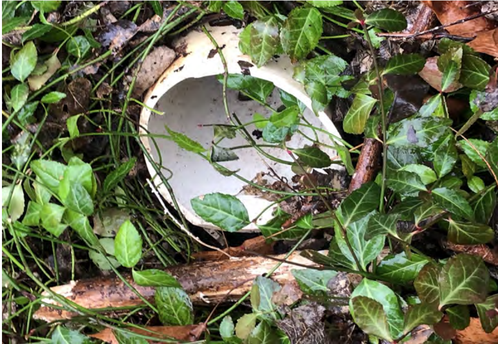
Photo 9: Photo of 6" drain pipe at bottom of sediment pond (notice broken riser).
